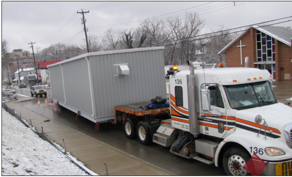
A fully integrated PanelShelter relay and control enclosure is delivered by truck
