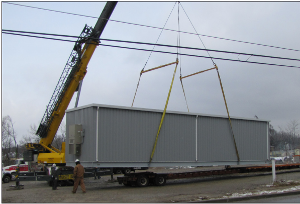
The relay and control enclosure is placed on piers
