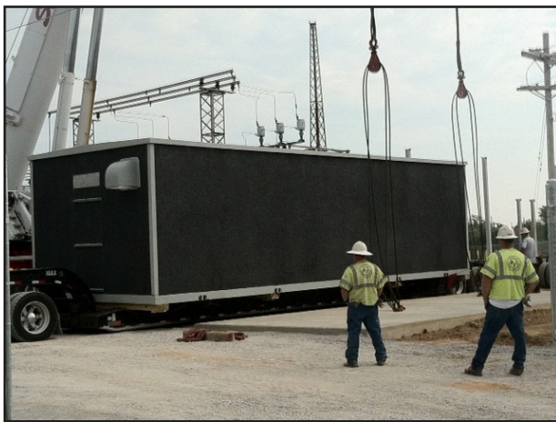
A concrete slab foundation was used in this application
