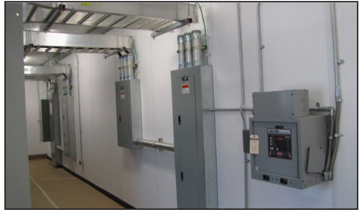
Pre-installed equipment includes batteries and chargers, HVAC, lighting, cable tray, transfer switches, AC and DC panels and more.
