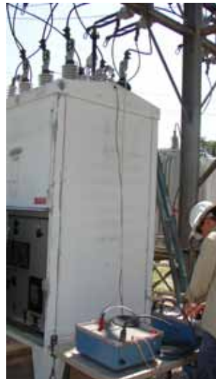
Hi Pot Testing a Vacuum Circuit Breaker
