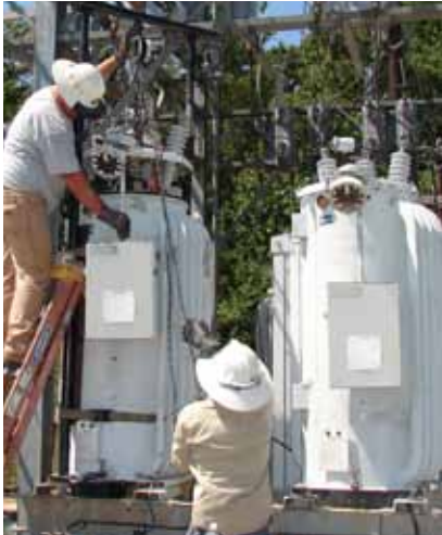
Removing the Top of a Regulator
