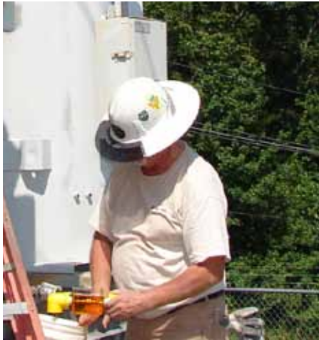
Oil Dielectric Testing
