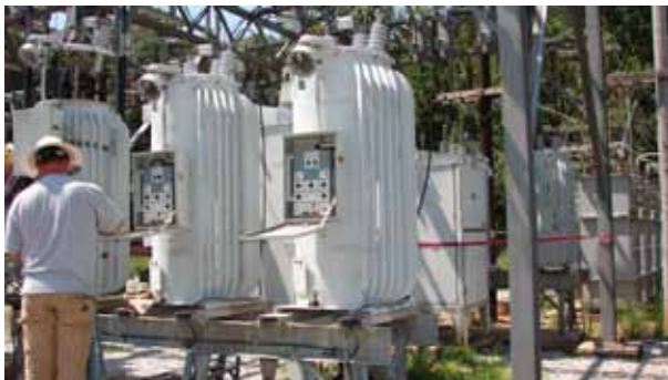
Testing Regulator Operations
