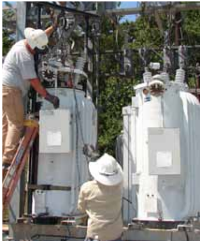
Removing the Top of a Regulator
