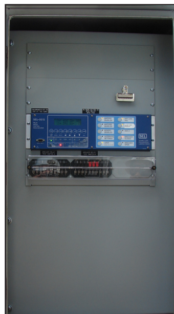
AFTER- Upgraded digital relays
