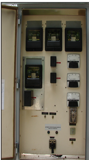
BEFORE - Relay Panel with old electro-mechanical relays
