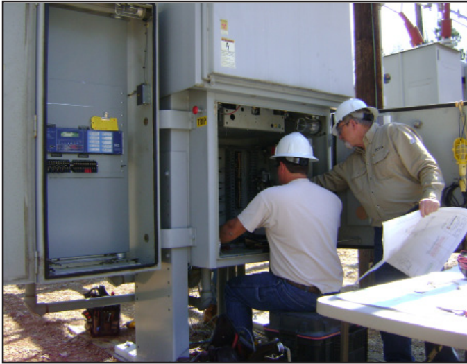
Installation of new Feeder Breaker Relays
