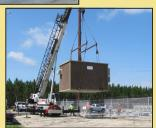
Metal or Concrete enclosures can be placed on piers, gravel or a concrete slab foundation. Larger buildings can be split into multiple sections for easier shipment.
