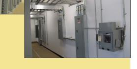
Pre-installed equipment includes batteries and chargers, HVAC, lighting, cable tray, transfer switches, AC and DC panels and more.
